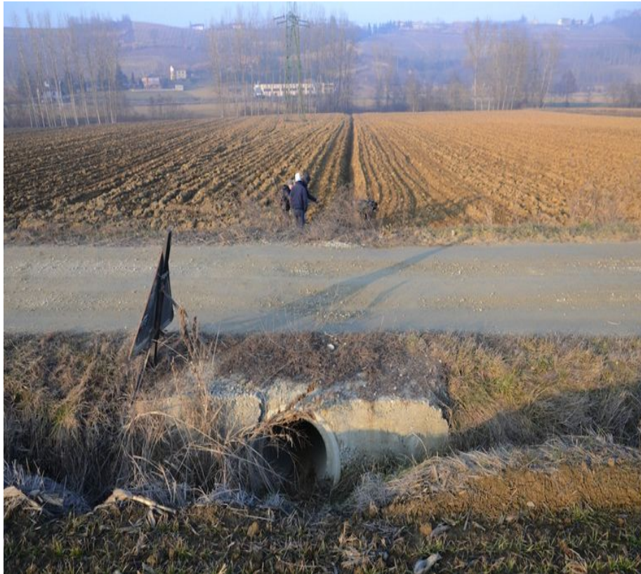
Picture: Pipe below road transfers runoff water fast via a deep furrow on the other side to the river
